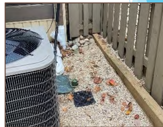
Unlisted Practice: Downspout Extension and Catch Basin
